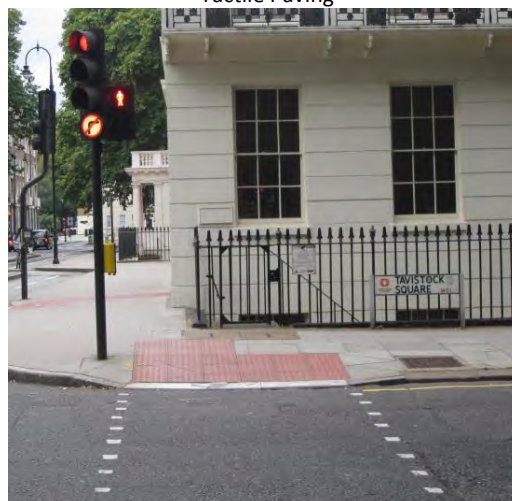
Figure 2.3: Pedestrian Crossing with Dropped Kerb & Tactile Paving
