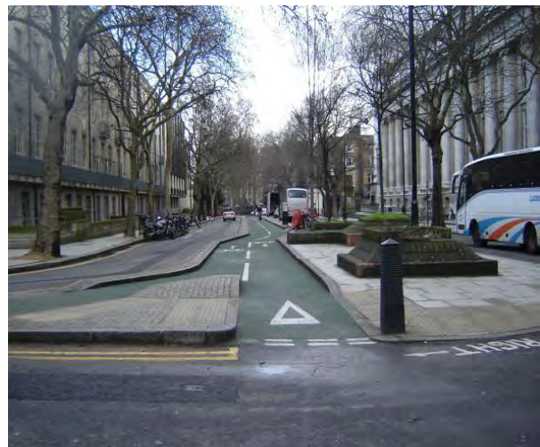
Figure 2.6: Segregated Cycle Track
